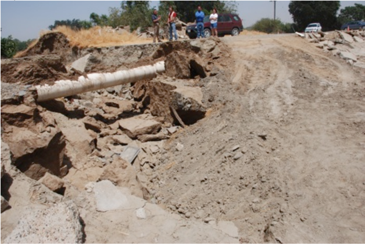
May 2008 washed out levee where over one million gallons flowed to Merced River
