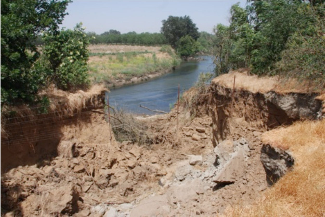
May 2008 Wash out of the banks of Merced River when over one million gallons flowed from a break at the Domestic Wastewater Treatment Plant
